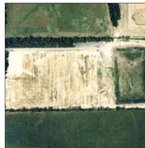
PAB Oil & Chemical Service, Inc. Abbeville, Louisiana
